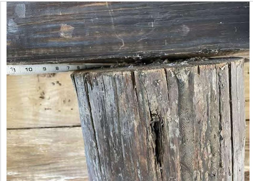
Abutment #1 pile E not fully contacting
