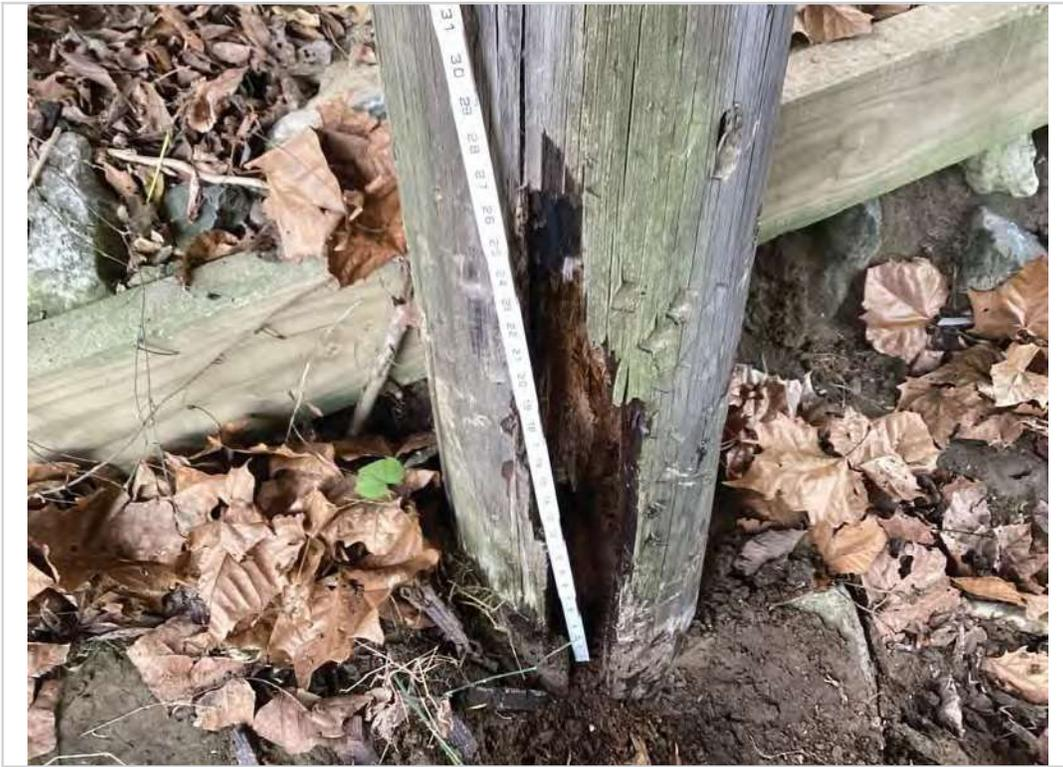
Bent 2 pile "D" decay
